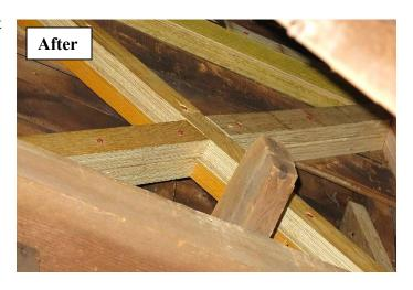
New hardware was installed to secure the new members to the existing structure. This hardware includes new hold-downs from the bottom of the rafter members to the stude at the belfry level, and horizontal ties at braces
